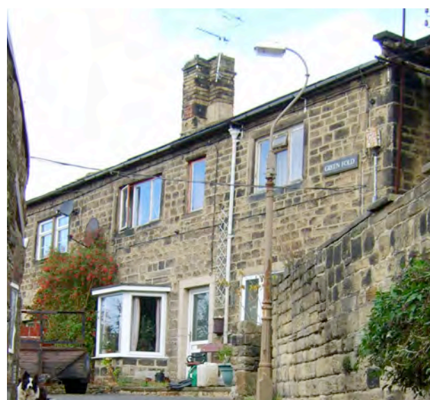
The alteration of openings, the removal of mullions and the installation of inappropriate modern style doors and windows is common in Baildon Green and detracts from the area's character.
