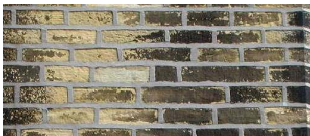
Example of a heavy, cement-based mortar used to point stonework. This type of pointing damages the stone over time and looks unsightly.
