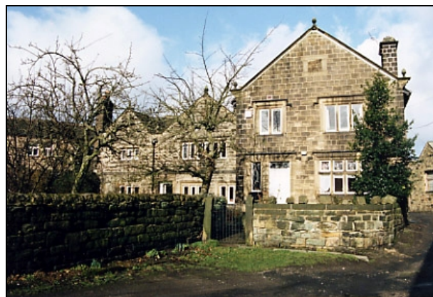
Old Hall, Westgate has a number of interesting stone features, such as kneelers and finials to the gable ends and hoodmoulds above the windows.
