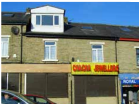
Vacant shops detrimental to the Conservation Area. Large dormer and fascias are inappropriate features.
