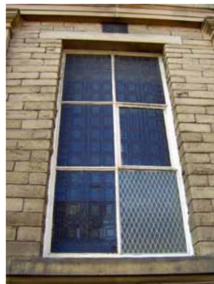
Above: Neglected windows with inappropriate window pane.
