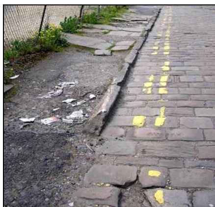
Darfield Street retains half of its settled surface, some stone kerbing and some stone flags, but much of these surfaces are in a poor state, particularly the pedestrian spaces.
