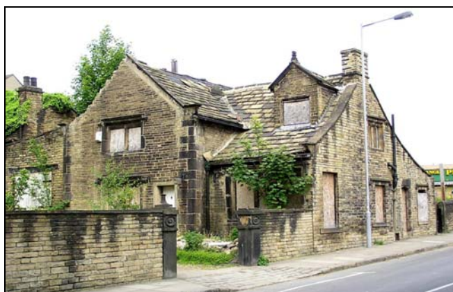
The Old Manor House has fallen into a very poor state of repair and urgent action is required to prevent further deterioration of its fabric.
