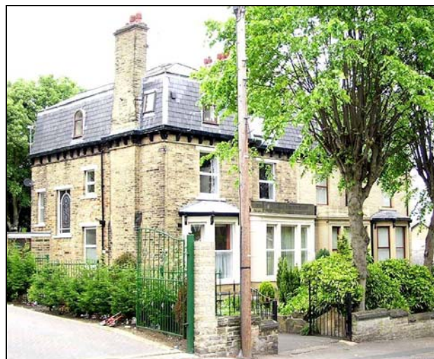
The mansard roof of 2-4 Park View Road is typical of later 19 th century houses in Manningham.
