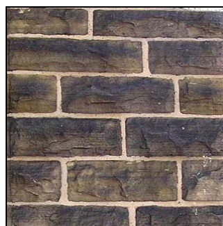
Coursed hammer dressed stone which has darkened with exposure to pollution and the elements. Note the traditional lime based mortar which is a lighter colour than the stone and is slightly recessed.
