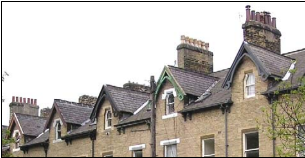
Slate roofs are an important and consistent detail for many buildings erected in the 19 th century. While the roof and dormer window detail in this picture are consistent, the missing chimneys spoil the roofline.
