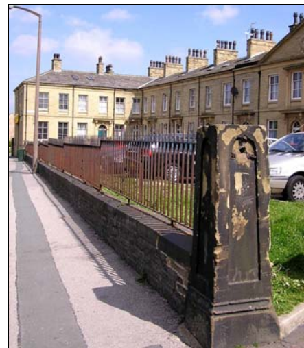
The iron railings remain attached to the shared boundary wall at Peel Square. The type of wall in this photograph is a typical boundary feature in Manningham. The damaged gatepier, the lack of paint to the railings and the pavement let this vista down.
