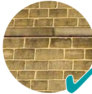
The mortar is of a sandy colour and texture and has been applied within the joints only to give a traditional look to the wall.
