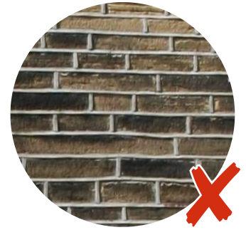
This smooth cement rich mortar contrasts with the stone of the wall. This is compounded by its application as strap pointing which stands proud of the stone.
