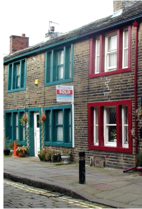
Traditionally all stonework, including the window reveals were left bare.
