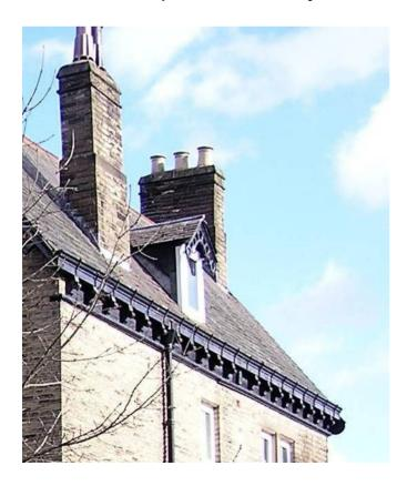
architecture in all types of building led to gutters being supported by stone corbels or brackets, often forming a decorative feature at the wall top, particularly at the houses of the wealthier classes, where the gutters would have a moulded (shaped) profile, while workers'
