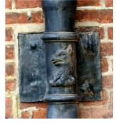
cottages or houses would have a more simply moulded timber gutter. There are some examples of housing built for the middle classes with moulded stone gutters with a lead-lined channel, and others with decorative hoppers and rainwater pipes, sometimes bearing a date or initials. The Arts and Crafts style of the late 19th and early 20th century saw a revival of the use of decorative moulded timber guttering in middle class houses.
