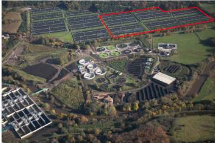
Photograph 1: Non-Operational Filter Beds at Esholt WwTW (development site location indicated in red).
