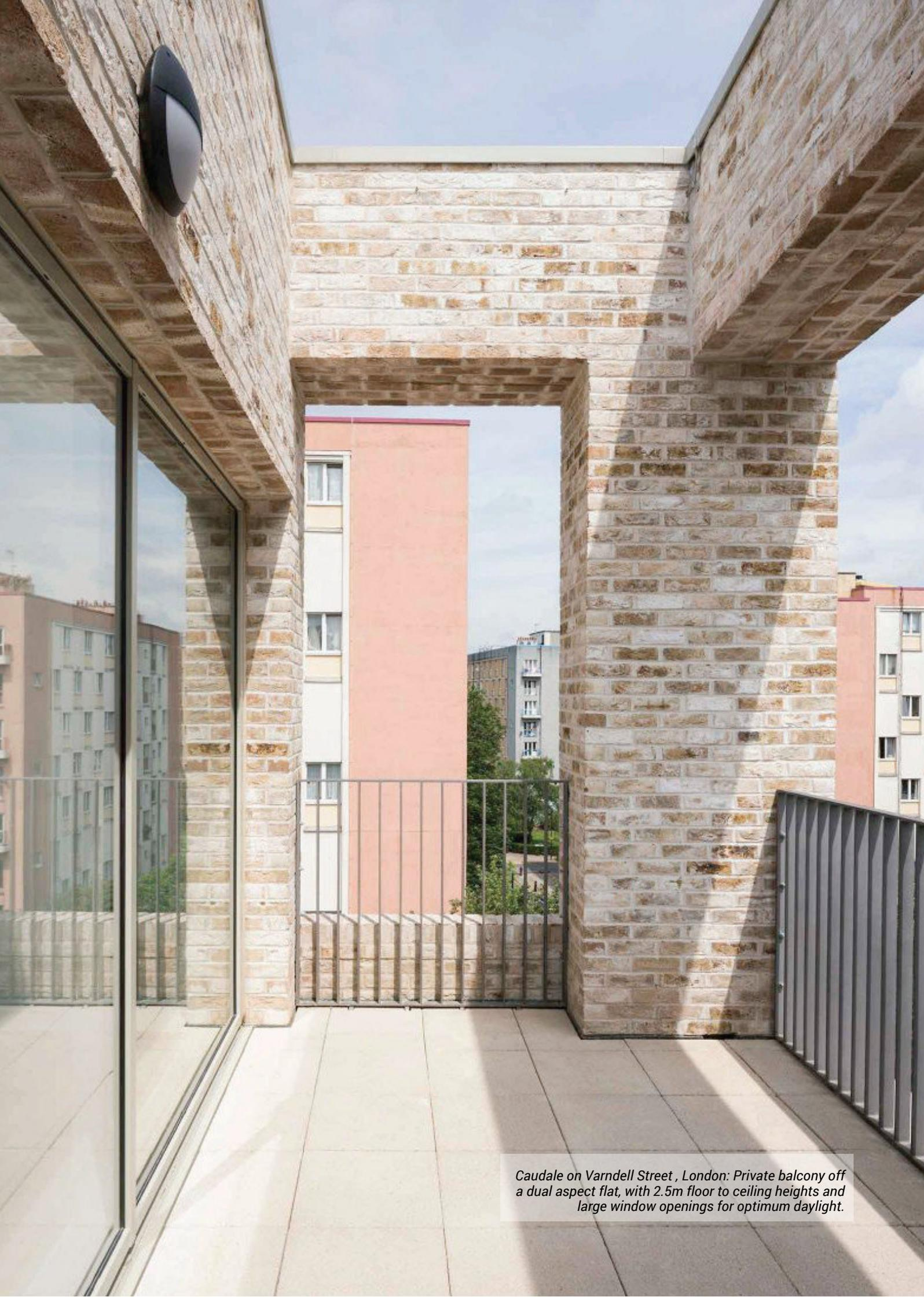
*Caudale on Varndell Street , London: Private balcony off a dual aspect flat, with 2.5m floor to ceiling heights and large window openings for optimum daylight.*
