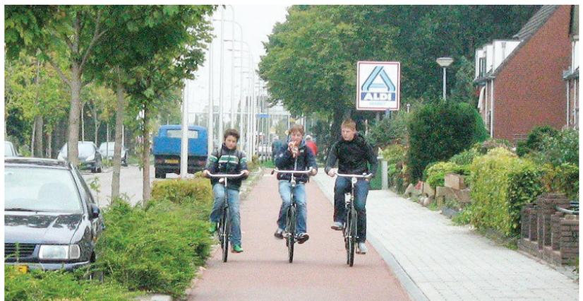
Separate cycle lanes, split from the road using planting and parking, create safe and easy-to-use cycle routes.
