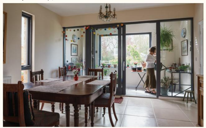
The Derwenthorpe development includes many innovative examples of energy efficient design. The homes have a highly efficient building fabric and are carefully orientated to ensure large windows face south to maximise solar gain. Many houses include sunspaces, offering a buffer between inside and out, collecting solar energy in the winter and cooling homes in the summer. Heating and hot water is provided from a biomass-fired district heating network which forms part of the development.
