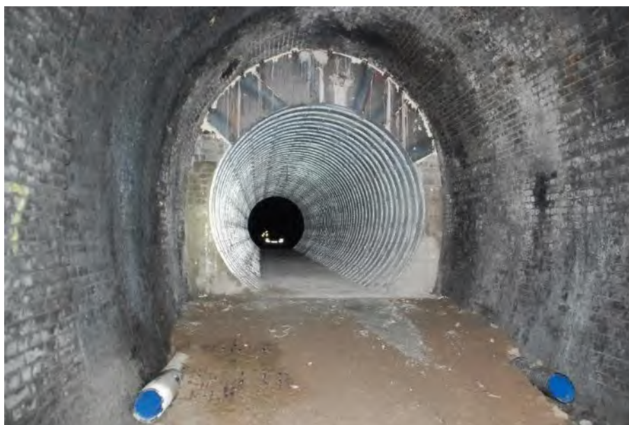
Figure 6: Corrugated steel pipe installed in Merthyr Tunnel.
