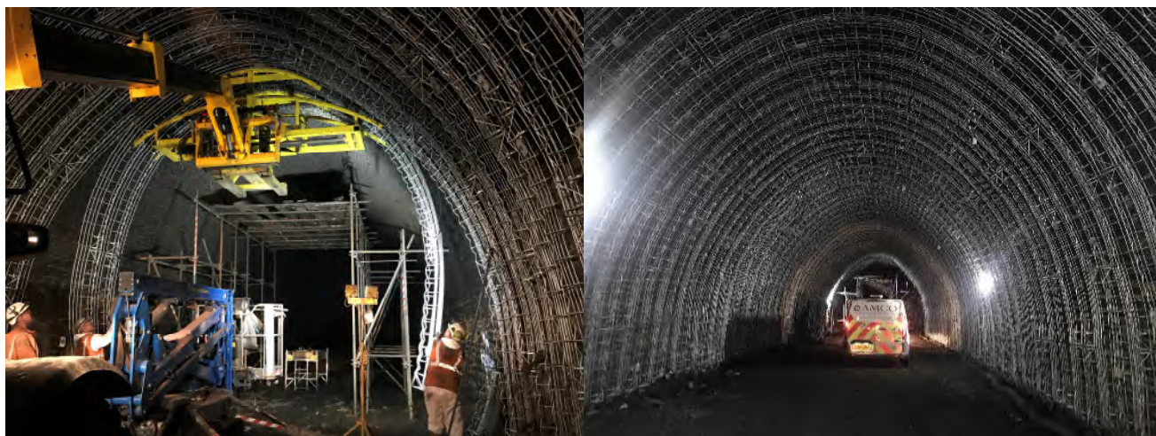
Figure 3: RAM Arch Installed at Queensbury Tunnel
