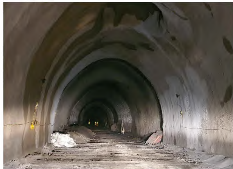
Photo 1: Typical example of spray applied concrete lining at shafts (Shaft 4)
