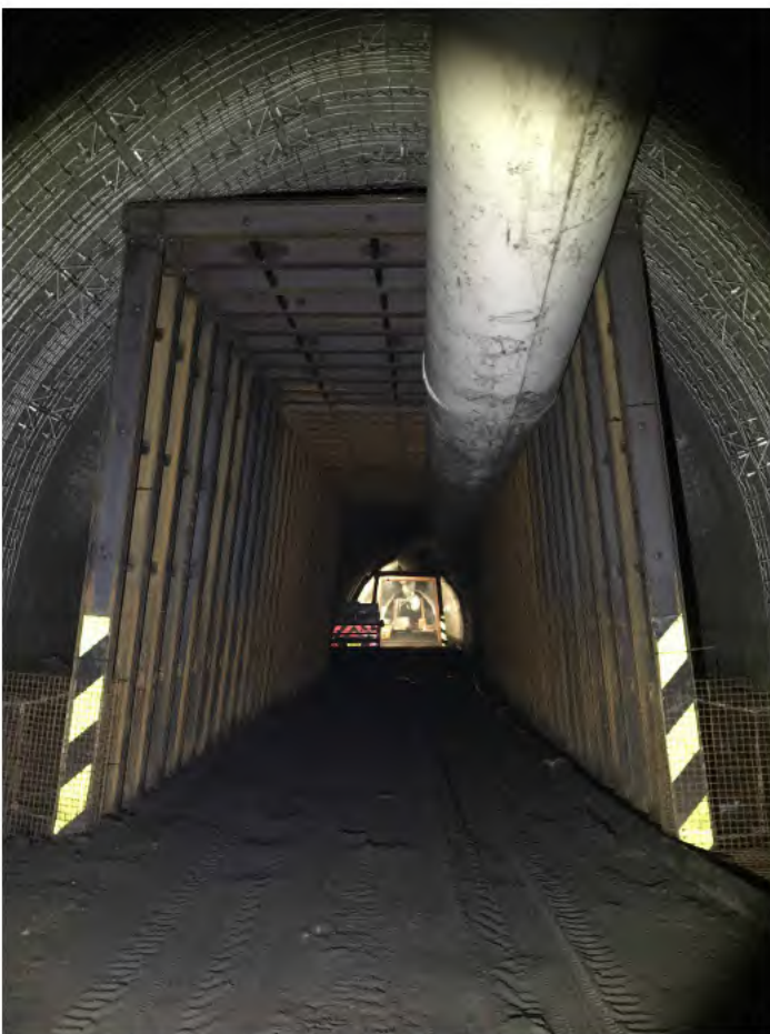
Photo 3: Example of Colliery Arches
