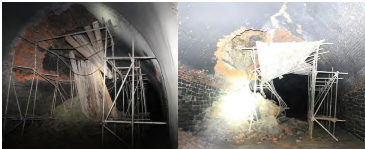
Figure 2: Collapses at tablets 90 (left) & 98 (right)
