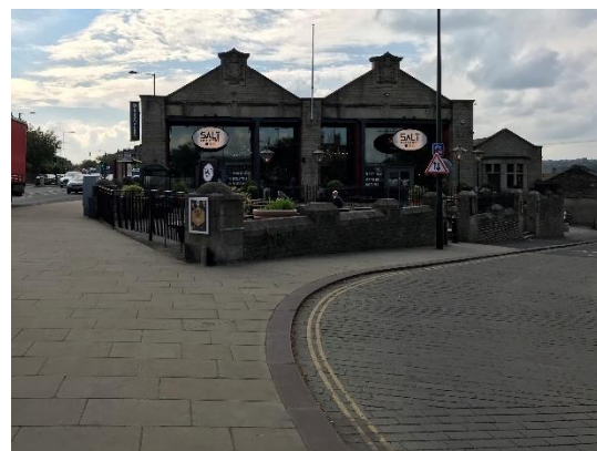
Former tram depot (Salt Bar & Kitchen) Bingley Road
