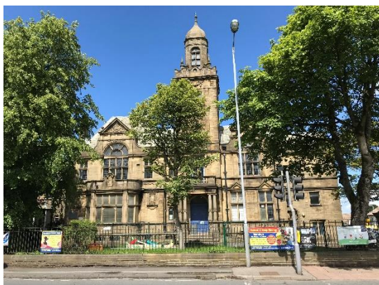
Queensbury Swimming Pool, Sand Beds
