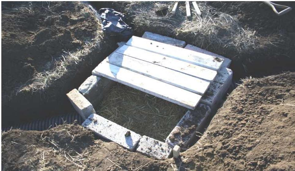
Figure 43 - breeze block chamber type otter holt constructed by Yorkshire Wildlife Trust with volunteers (courtesy of Don Vine)
