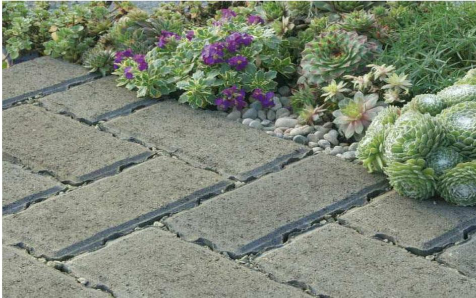
Figure 69 – an example of attractive permeable paving in use on a driveway (Luxury Paving, no date)
