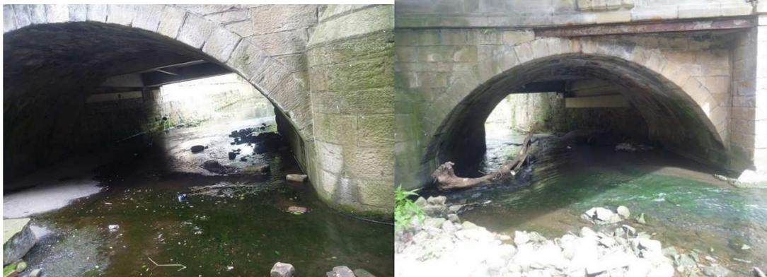
Figure 36 (left) - western tunnel & Figure 37 (right) eastern tunnel, both under Briggate A657 road-bridge with partial concrete and stone-lined beds
