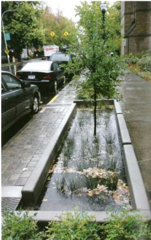
Figure 66 – infiltration stormwater planter in which intercepted rainwater will either filter down through the soil and infiltrate the ground beneath or spill over into the adjacent drain (photo by Tom Liptan).
