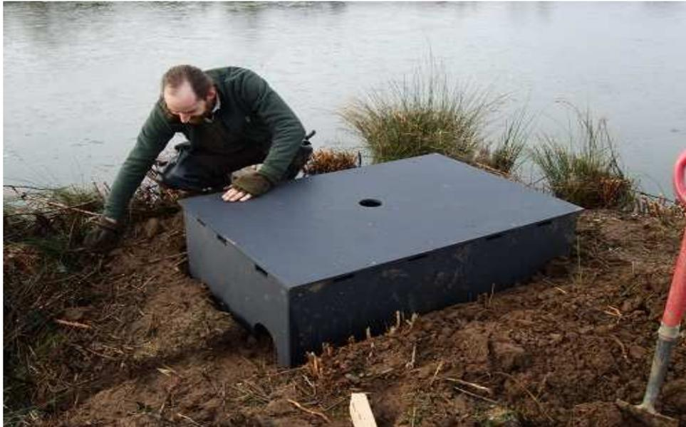
Figure 42 - recycled plastic chamber otter holt comes flat packed. Installed by Yorkshire Wildlife Trust and volunteers (courtesy of Don Vine)
