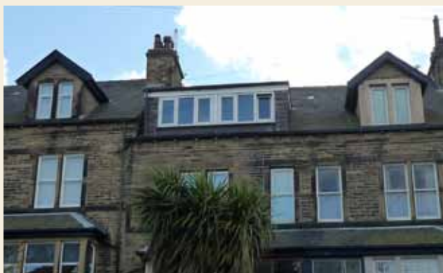
Figure 38: Unacceptable - original dormers should not be replaced by box type dormer windows
