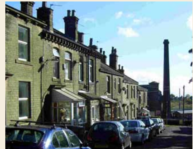
Figure 26: Porches can damage the streetscene
