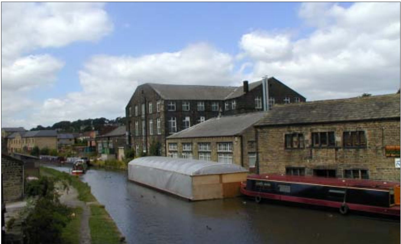
View westward along the canal
