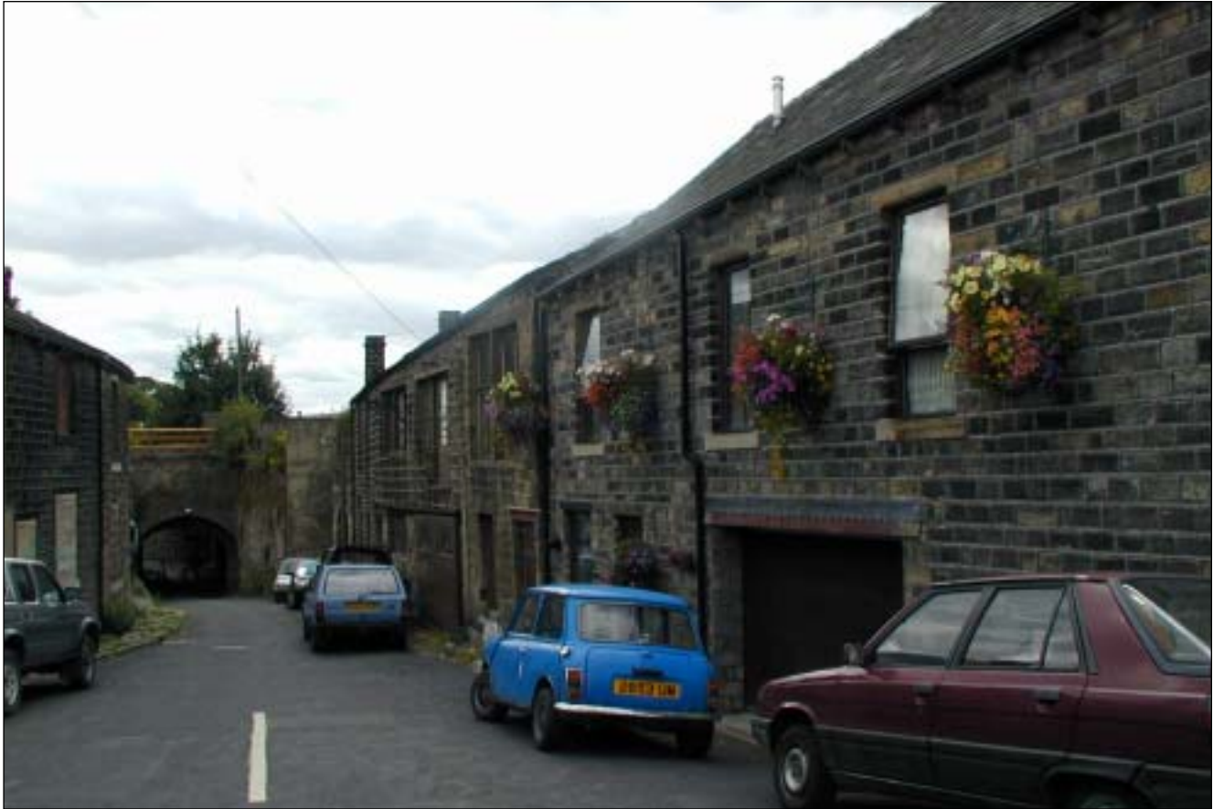
View down Hainsworth Road to the Aqueduct (Grade II) – an attractive street, although part of it is in a semi-derelict state. This is a traditionally industrial part of the settlement: a forge has been on the site of one of these buildings for over five hundred years.
