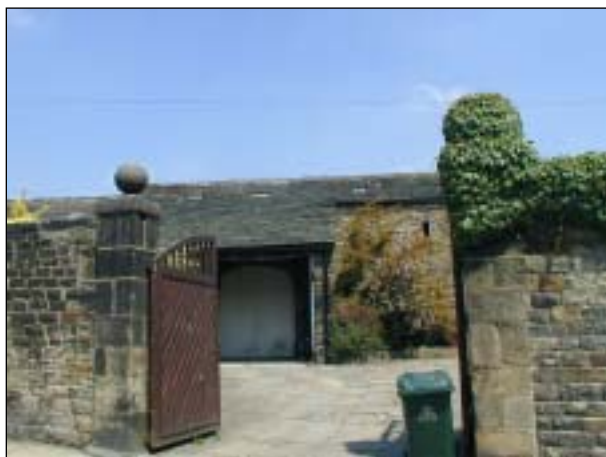
Barn associated with Old Hall Farm (Grade II) – the quality of this area is outstanding.
