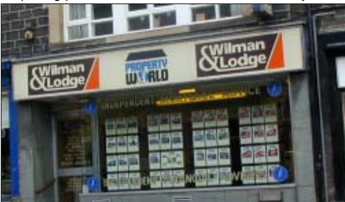
Example of a poorly detailed shop front on Kirkgate, the materials, scale and detail of which is not complementary to the building on which it is situated or the character of the street.
