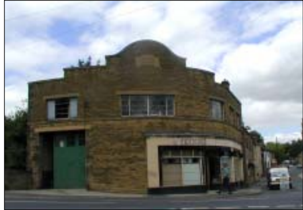
The Co-op building (unlisted) – constructed in the 1930s and Art Deco in style.
