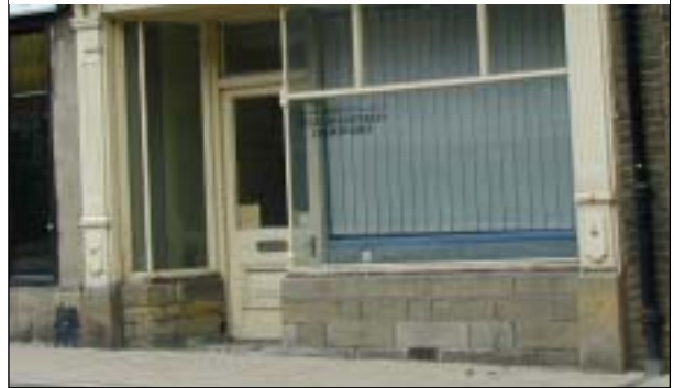
Example of a well designed traditional style timber shop front, with its characteristic cornice, consoles, transoms, pilasters and stall riser. The detail is complementary to the building on which it is situated and adds interest to the street
