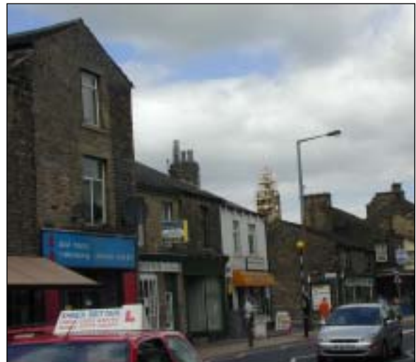
Varying roof heights of the retail premises of Kirkgate, creating an intricacy of form.
