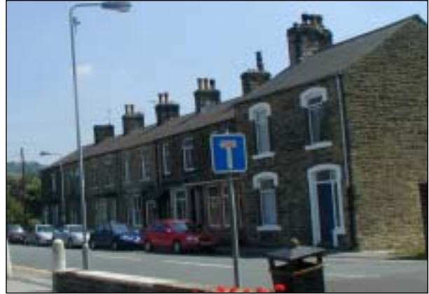
Terrace buildings of Wesley Place (unlisted) – they are typical of the area being constructed of local stone with slate roofs.
