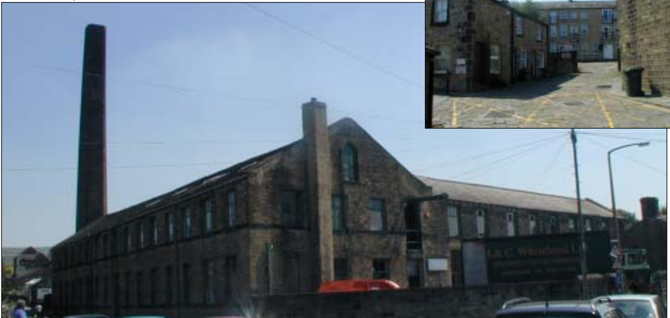
Waterloo Mill – The only Grade II* building in the conservation area and Airedale Mews (unlisted).
