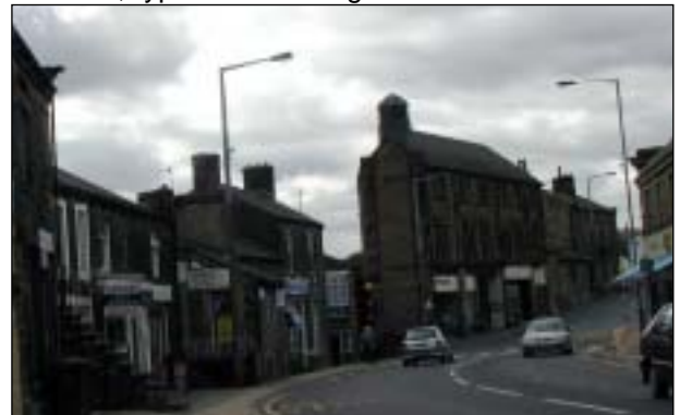
The Co-operative Society building (unlisted) – unusual in design and situated at a prominent terminal point of Kirkgate
