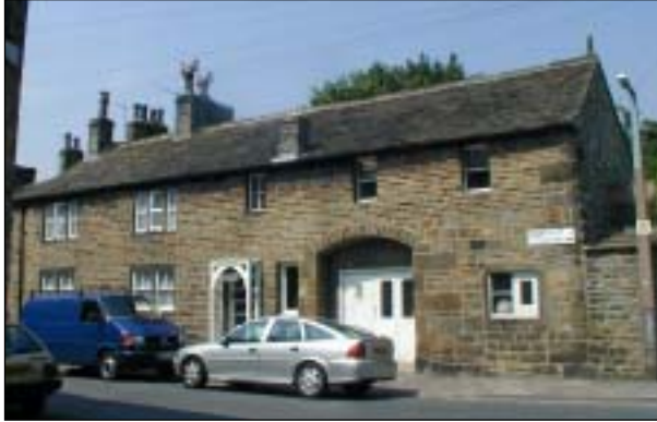
27 North Street (unlisted) – a former laithe house, with characteristic wagon entrance and a stone slate roof.
