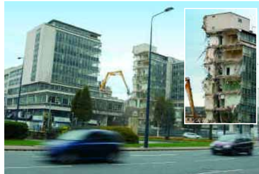
Nibble by nibble the jaws of a 100-foot crane have eaten into Forster House as demolition makes way for the Broadway development in the city centre.
