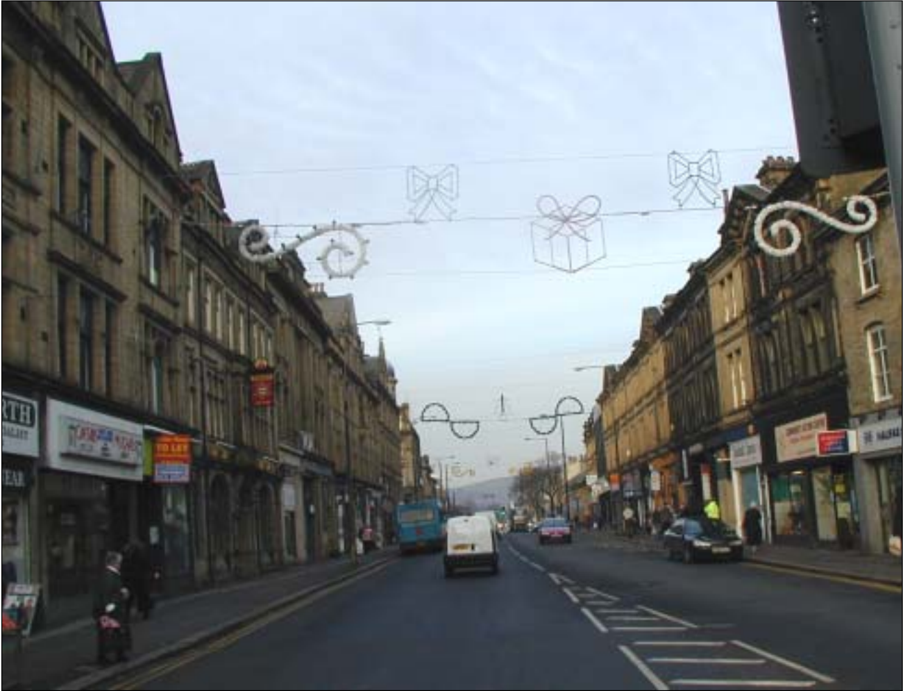
The wide North Street, with its ornate commercial premises, many of which are marred by poorly designed shopfronts and fascias.
