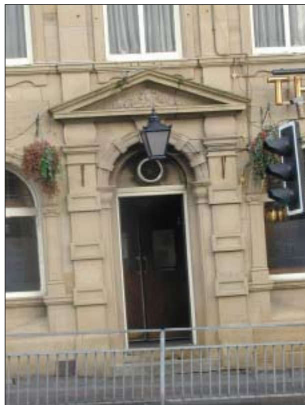
Doorcase detail of Cavendish Hotel
