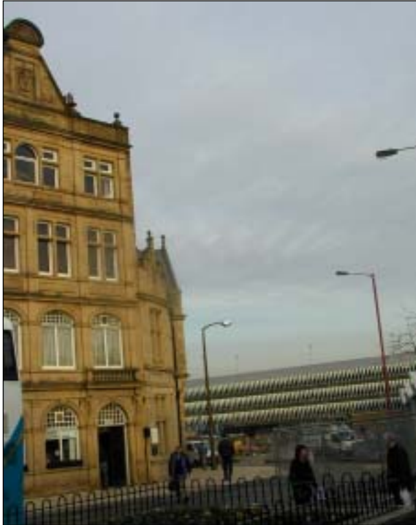
Juxtaposition of the old and the new along the Lawkholme Crescent boundary of the conservation area
