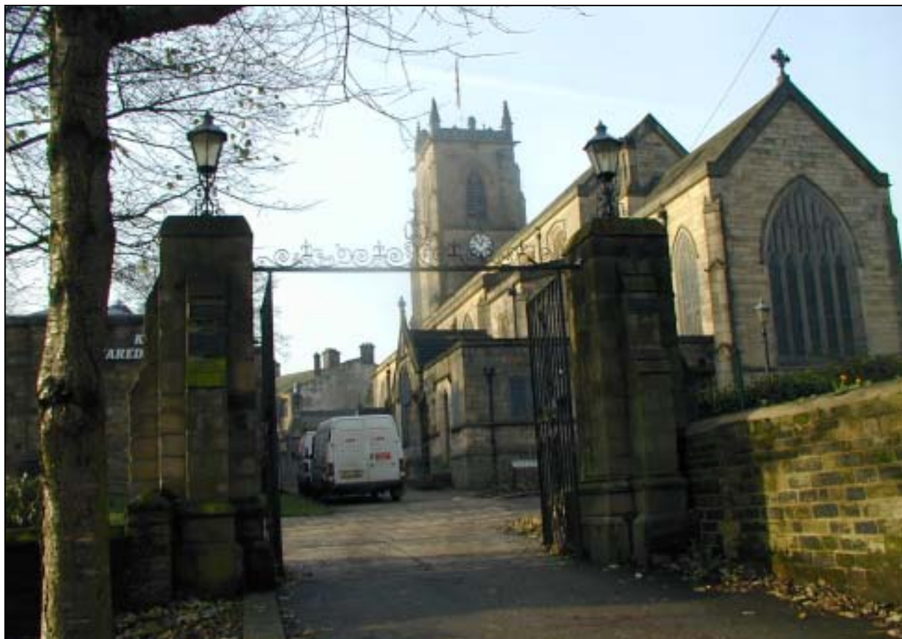
Rear of the St. Andrew's Church (Grade II) from Market Street, with ornate entrance gates
