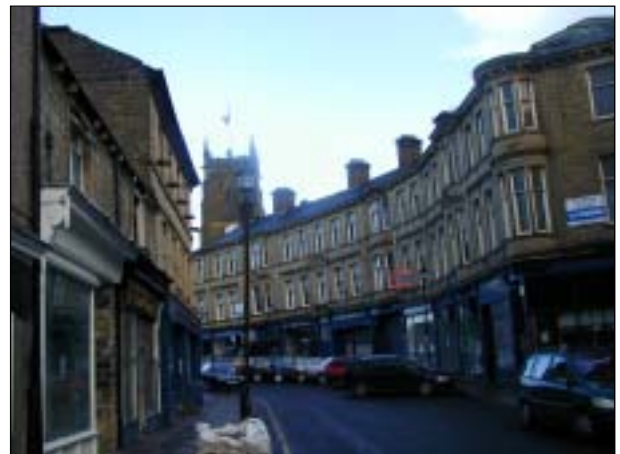
Hattersley's Crescent (Grade II), Church Street
