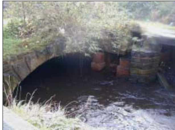
Old bridge over North Beck
