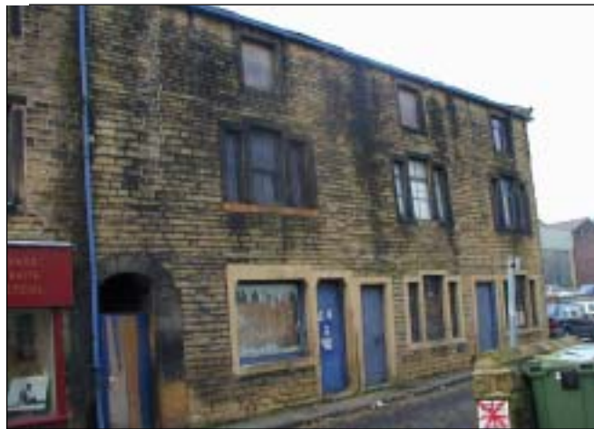
7-9 Chapel Street (Grade II)
