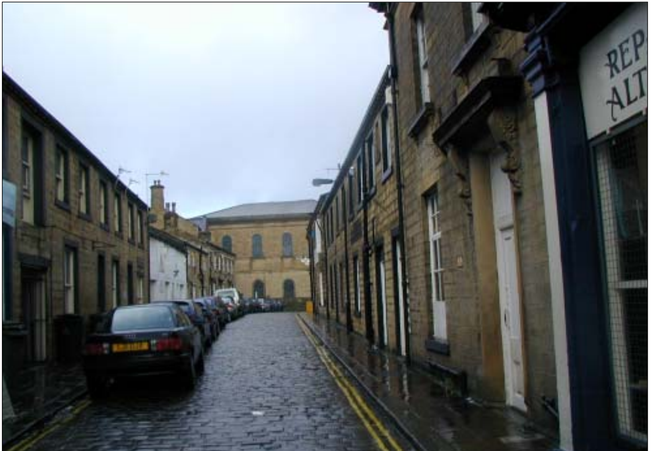
View down Temple Street from High Street – characterised by two storey simple buildings and narrow setted street. The Grade II listed Mosque, originally a Methodist Church constitutes the terminal focus of the street.
