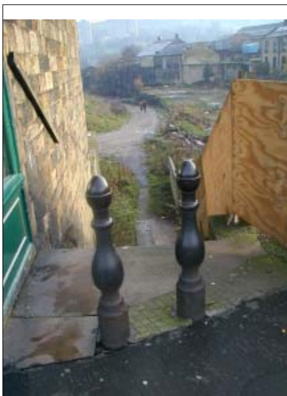
Early cast iron bollards, Water Lane
