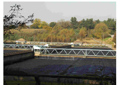
Esholt sewage works
