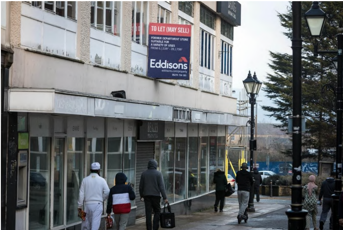
Figure 1-16 - Vacant former Beales store on Low St 31
