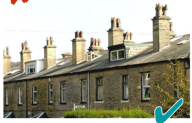
Top: Only two of the nine houses in this terrace retain all their details giving a disjointed skyline. Above: The retention of full height chimneys and pots gives this terrace a uniform appearance.
