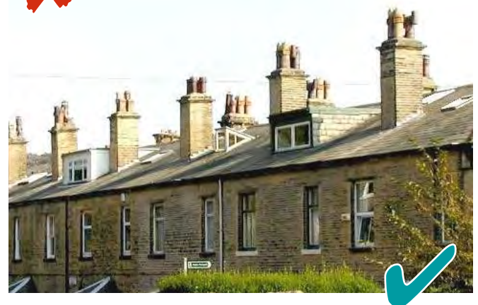
Top: Only two of the nine houses in this terrace retain all their details giving a disjointed skyline. Above: The retention of full height chimneys and pots gives this terrace a uniform appearance.
